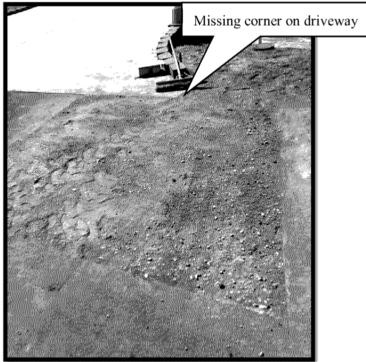
Picture of Repair as of 4/7/2020
